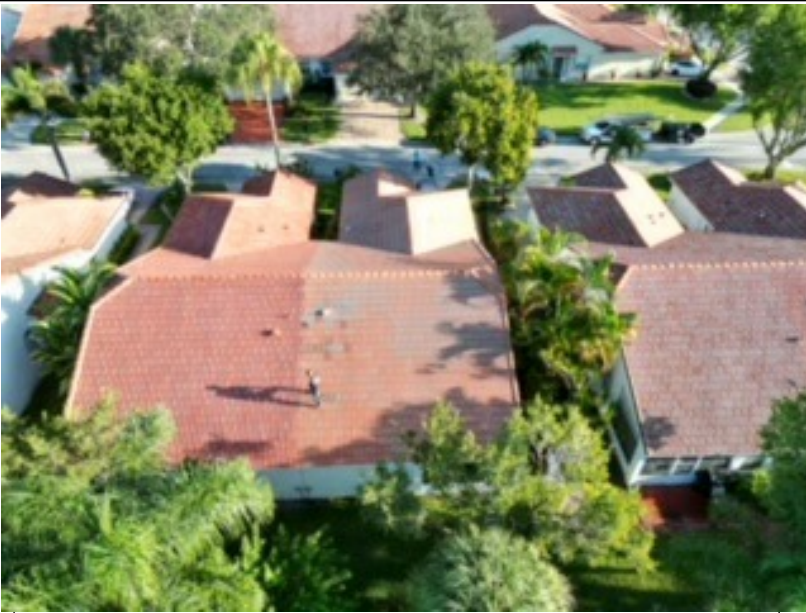
Aerial view of roof covering
