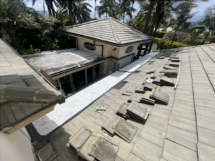
New underlayment and flashing systems installed, existing tiles reset, and roof returned to serviceable condition.
